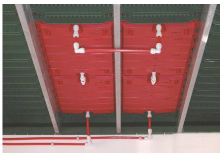
Fig. 12: Thermo W connection with the connector system
