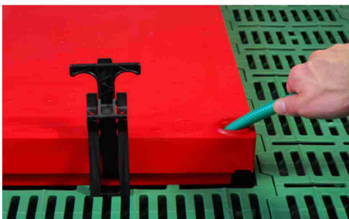
5. fill panel pressureless with water hose
